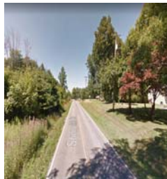
Figure 19F: Sunnyside Road looking north
