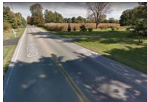
Figure 23E: Bogart Road looking east
