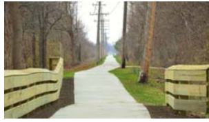
Figure 16E: Lake Erie Electric Rail Trail
