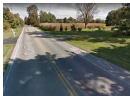
Figure 20E: Cleveland Road looking east
